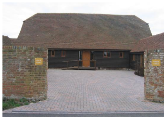
East side to courtyard.
