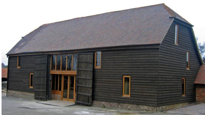
West side and main entrance
